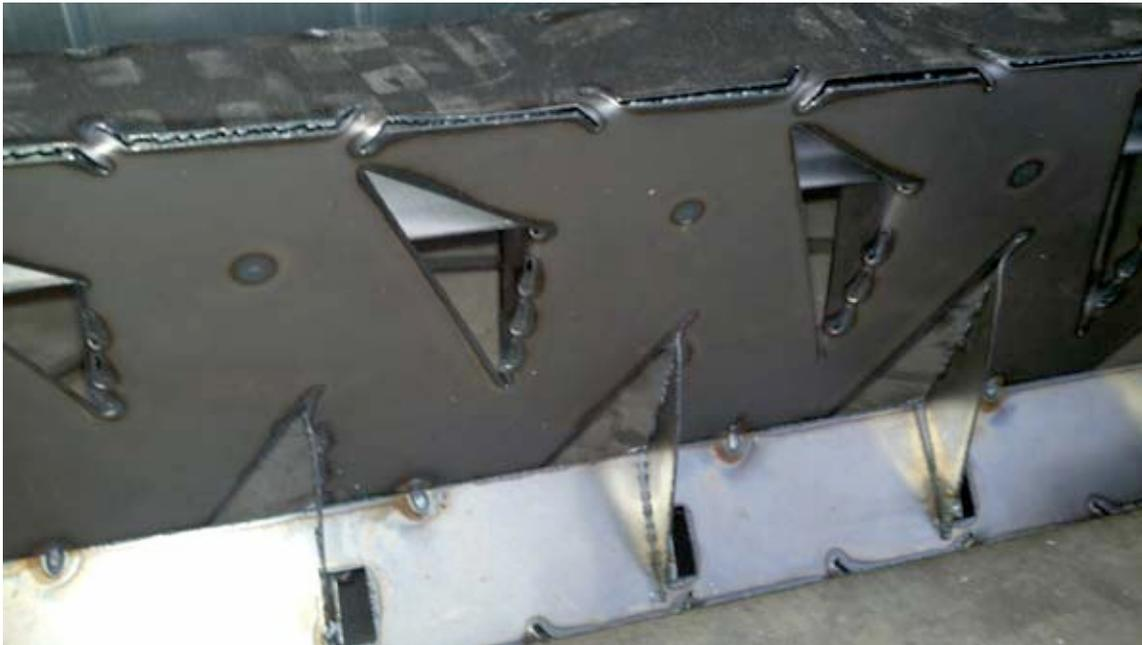
**Figure 18. An additional tack weld was necessary between webbing fins to keep the chord rigid.**
